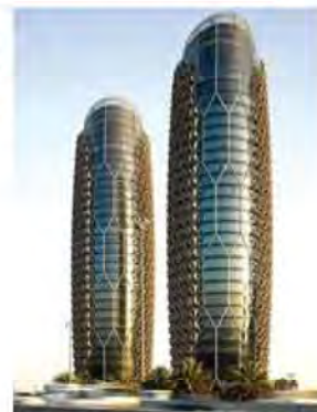
Al Bahar Tower, Abu Dhabi.
